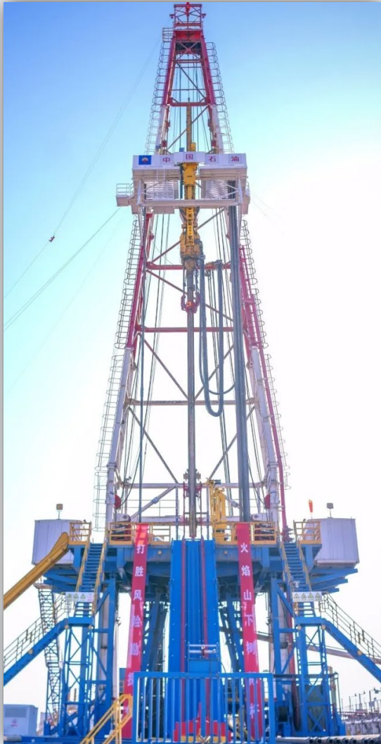
Triprio @ XD 70202 Rig
